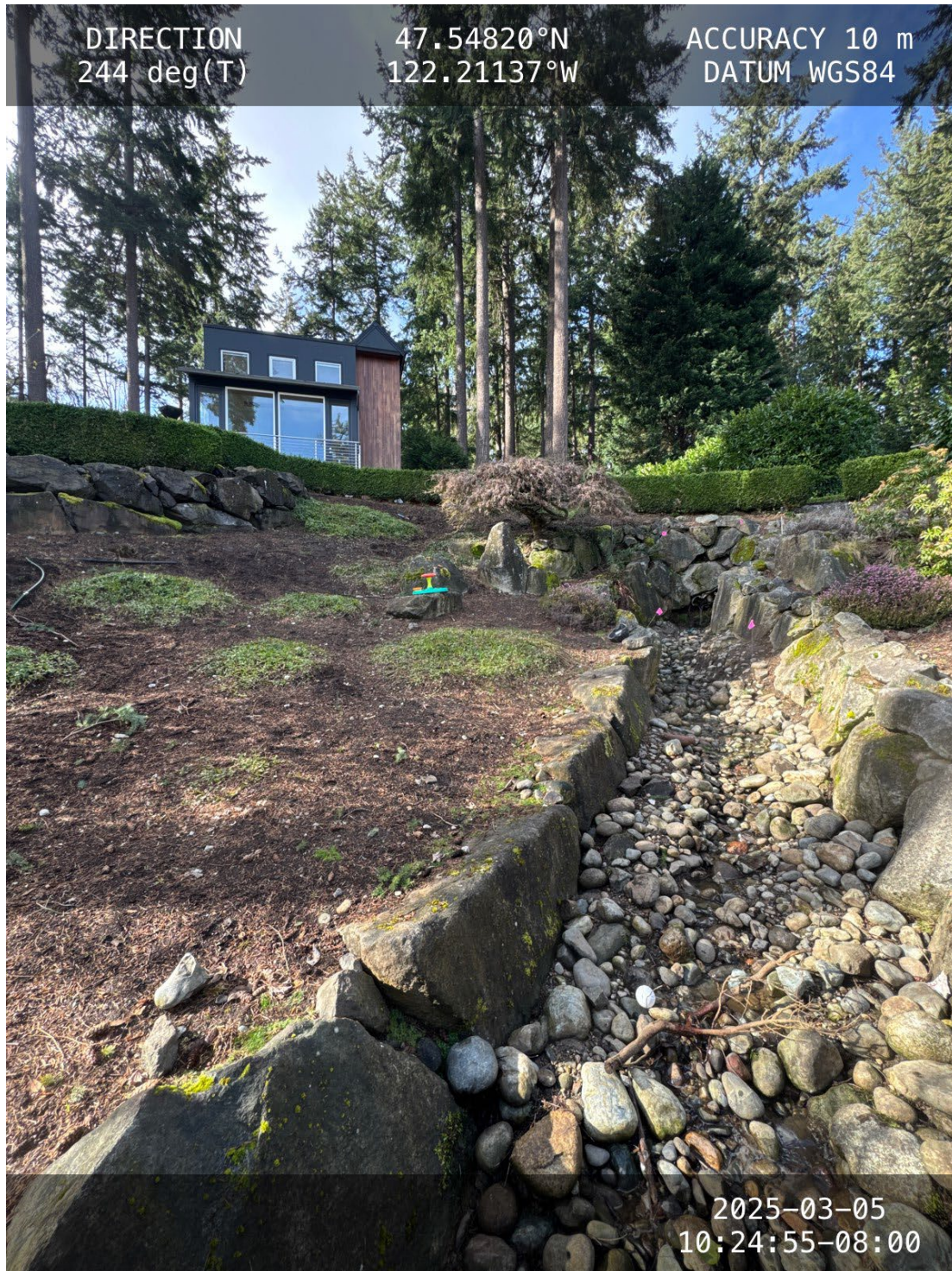
Photo 1. Photo of onsite watercourse (Stream 1) located within created rock channel that continues offsite through a pipe to the east, photo taken facing upslope to the west toward house.
